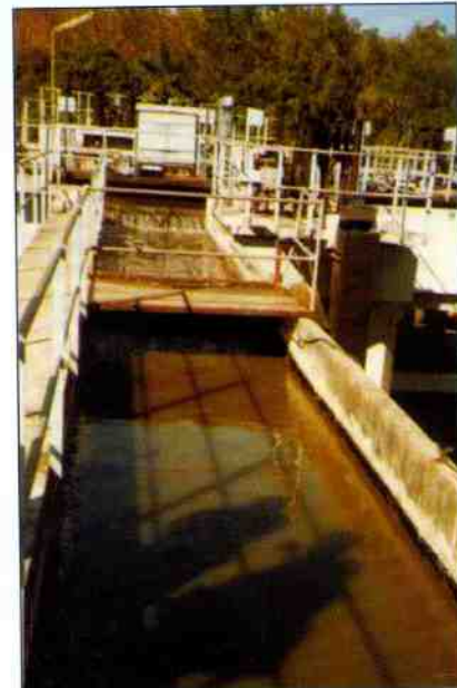
UASB Sewage Treatment Plant at Kankhal (Hardwar)
