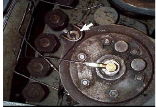
Fig.7 shear pin detector in guide vane arm
