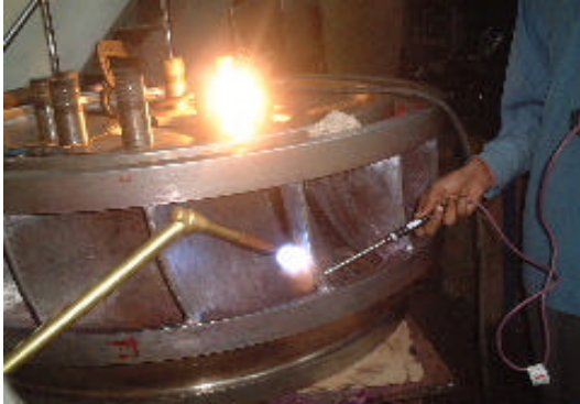
Figure 5. Runner preheating
