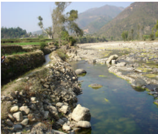
Figure 3.1 downstream irrigation canal
