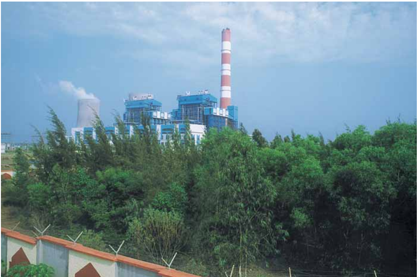
A coal based power station - Simbadri
