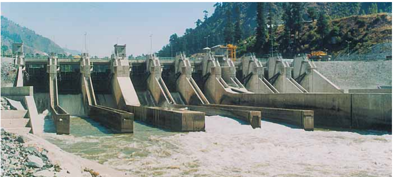
Barrage of Hydro Power Station - Uri
