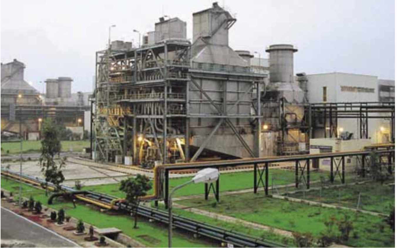
Gas Based Power Station - Auraiya
